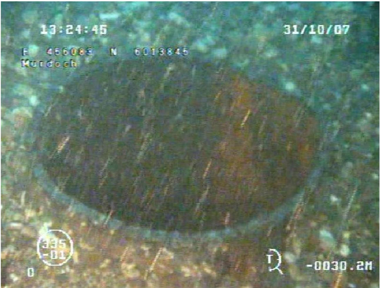
Figure 3.4.1: Residual pile stick-up prior to installation of mattress
