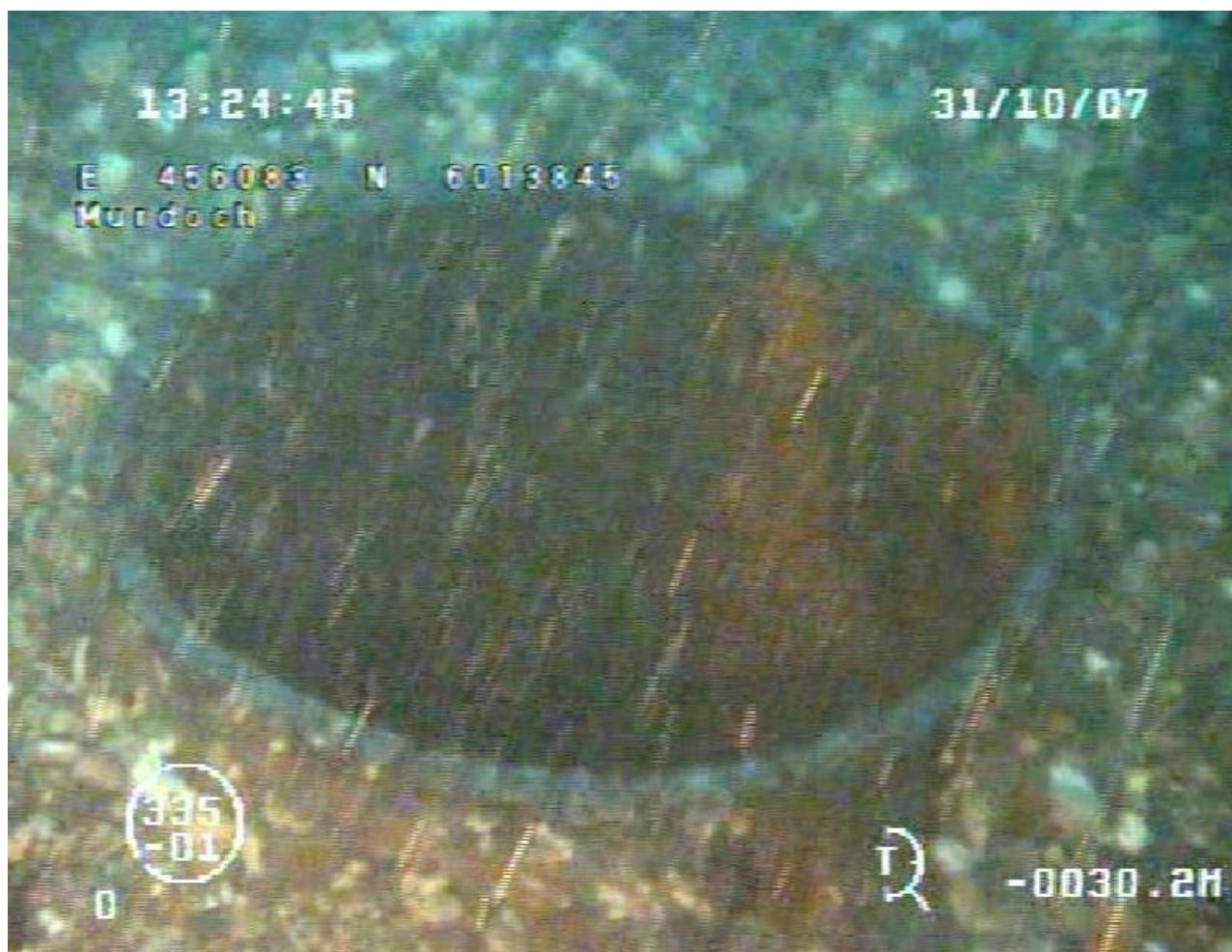
Figure 3.4.1: Residual pile stick-up prior to installation of mattress
